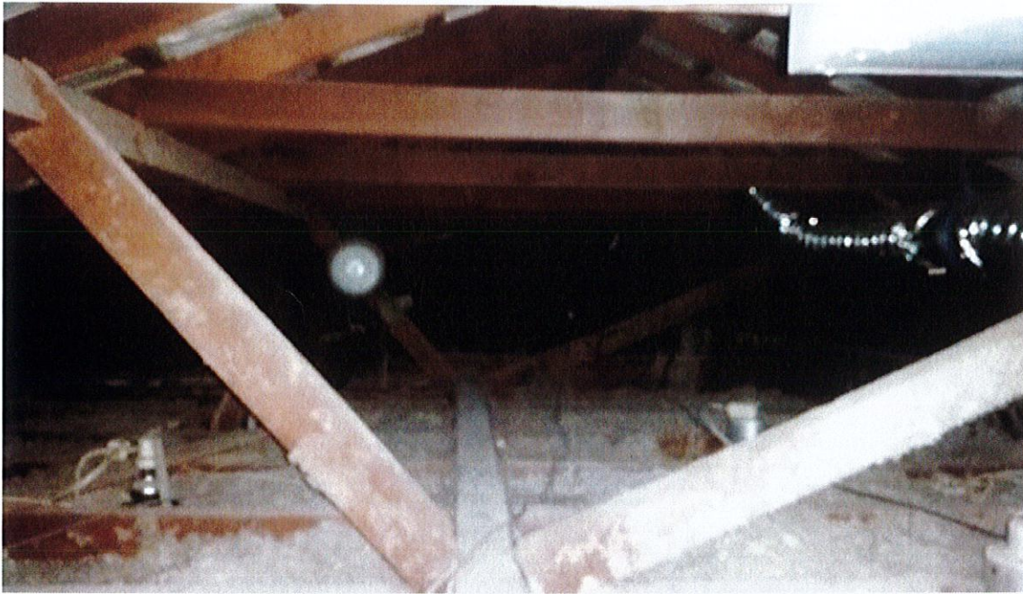
Photograph 1: Representative photograph of ceiling space
